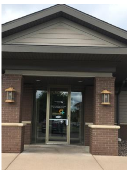
PHS Building- 4252 Southtowne Drive Suite C Eau Claire, WI
